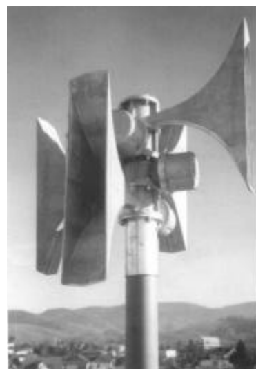
Siren system in Bühl (Germany)
