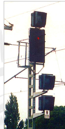
Exit signal (Ks) with auxiliary signal indicators
